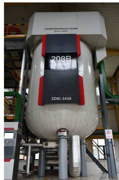
Submerged Electrode Steam Boiler
