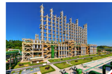
Distillation tower for high-purity polysilicon of Yongxiang Co., Ltd.
