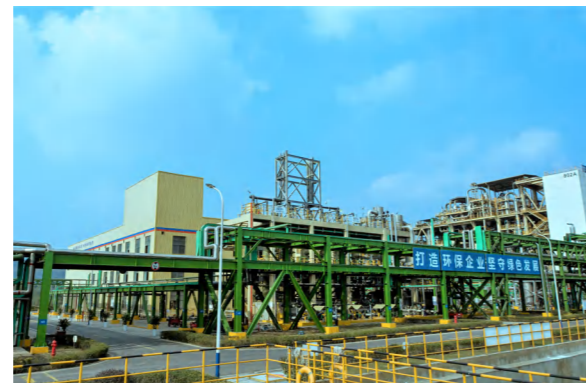
Wastewater Treatment Station/Technical Treatment Process
